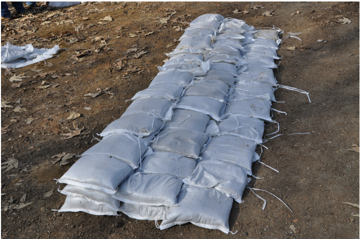
Sandbag Wall Construction
