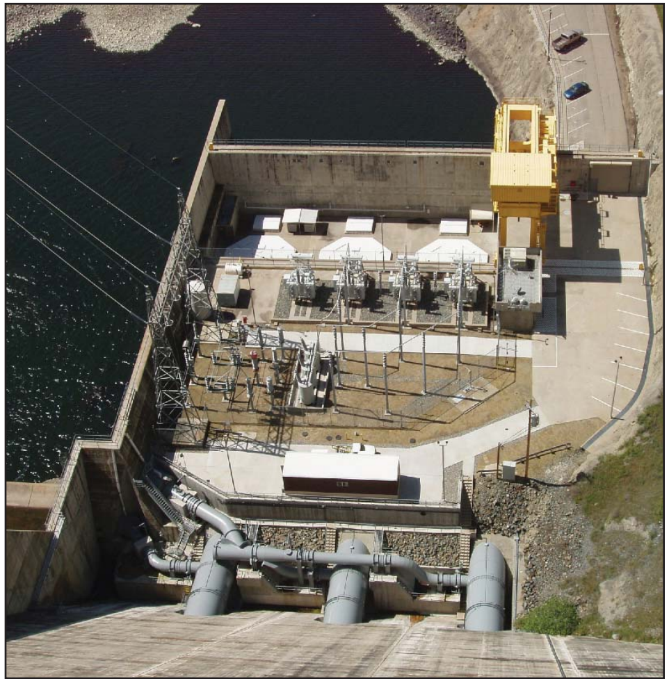
Looking down from the top of the dam at the Jeff L. Taylor-Pine Flat Power Plant. The large pipes emerging from the dam are penstocks carrying water to the turbines. The smaller pipe system at the dam's base is part of the new turbine bypass.
