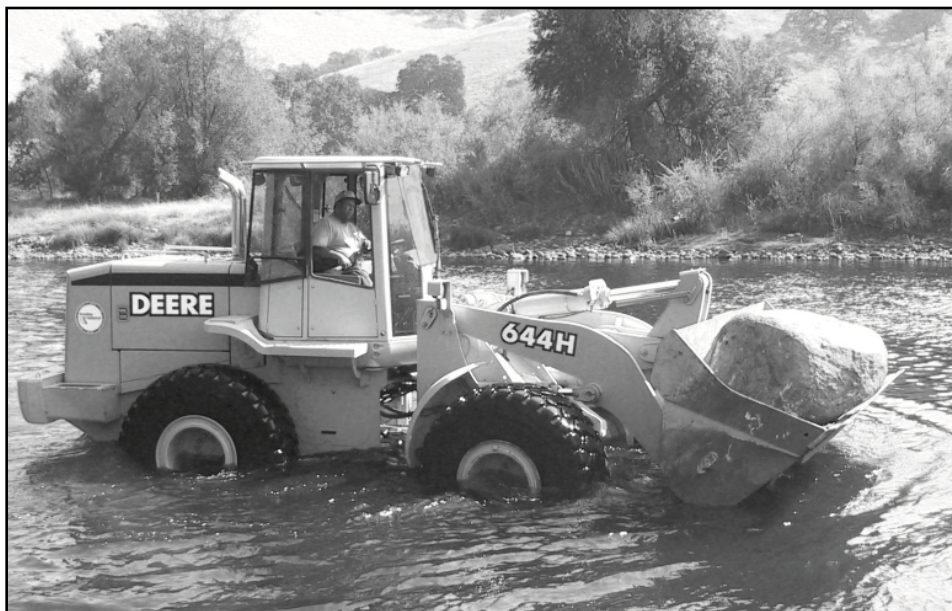
Boulders by the thousands have been placed in the channel for enhanced habitat under the Kings River Fisheries Management Program.
