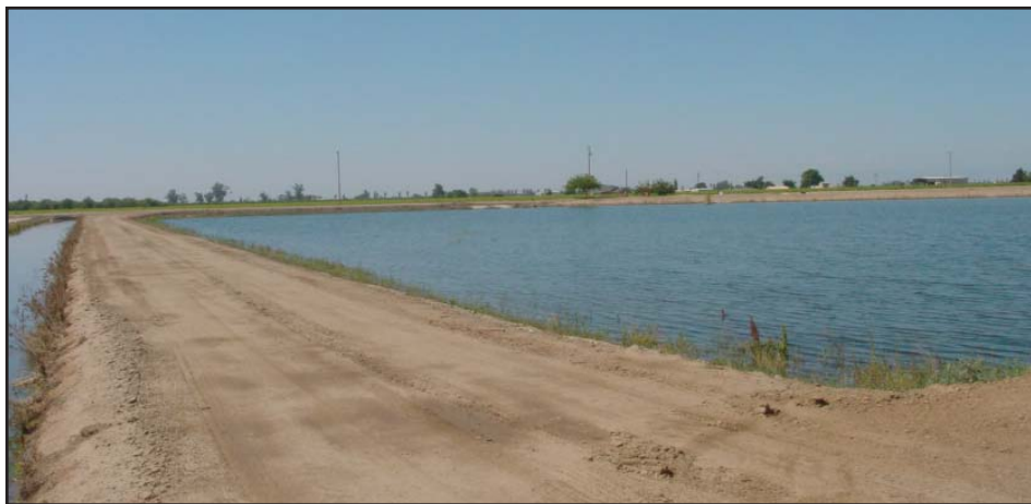
The Waldron banking facility is an example of an effective partnership between the Fresno Irrigation District and the City of Clovis, and how new water projects can be developed.
