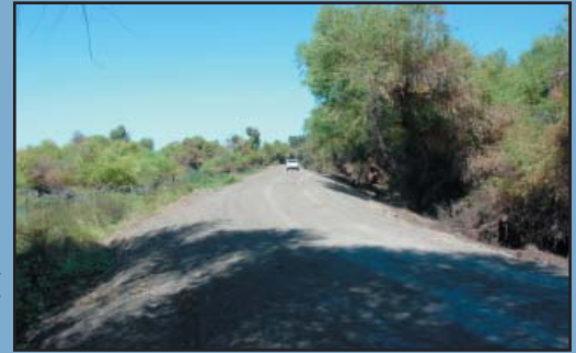
Same area as above, after clearing and grading.
