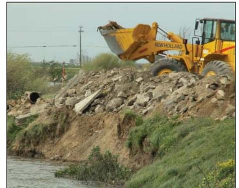
*A skip loader places rubble along the bank of the North Fork of the Kings River for protection from additional sloughing.*
