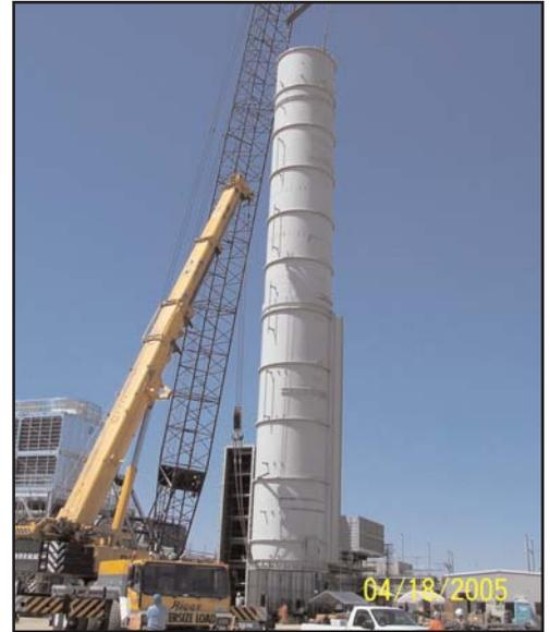
One of two 120 foot tall stacks is erected using one of the largest cranes in the region.
