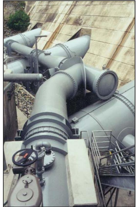
*The Turbine Bypass pipelines link and span the Pine Flat Power Plant's three penstocks at the base of Pine Flat Dam.*
