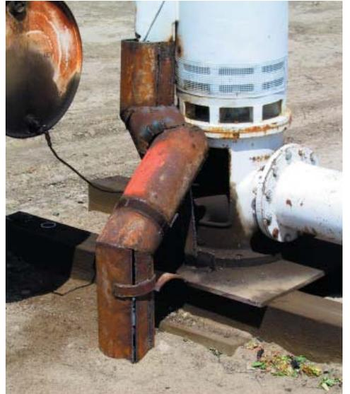
Figure 2. An example of grower-built wire protection.
