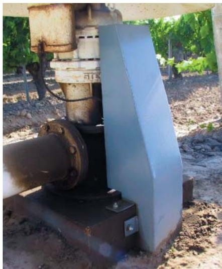
Figure 1. An example of pump company built wire protection.
